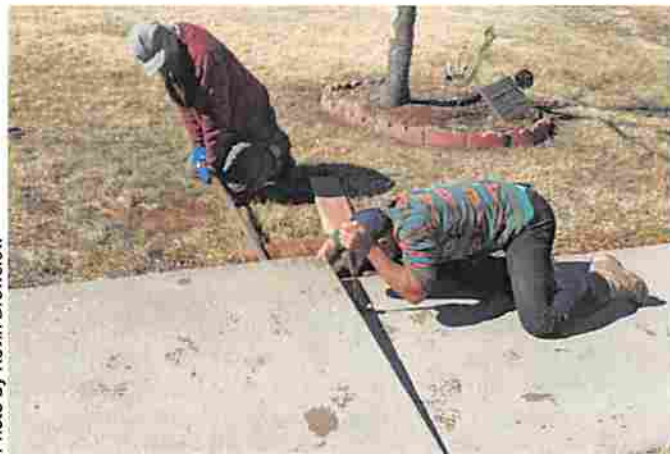
Danny lifts the slab so Luke can install a shim
